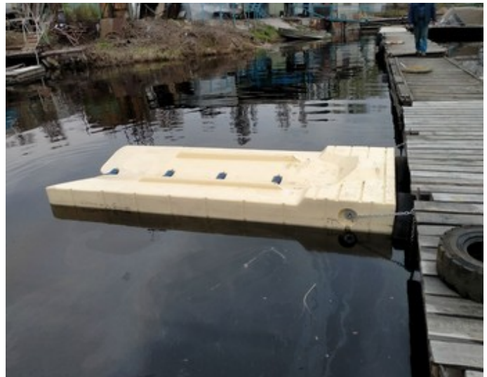
Jet ski connected to fixed/floating pontoon
