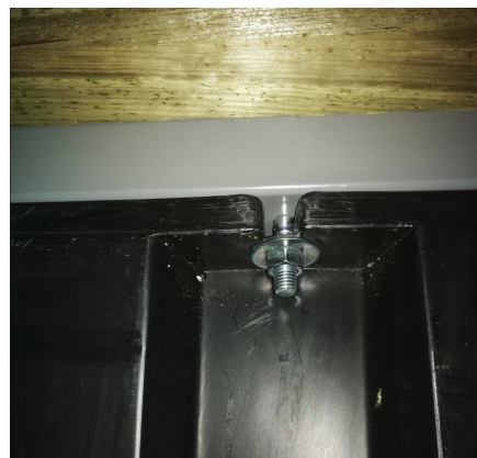
Connection of float to Steel frame
